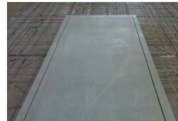
FIGURE 8 Saw kerfs for rodding
