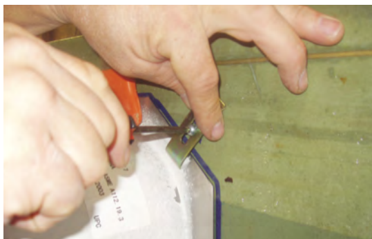
FIGURE 9 Undermount sink mounted with mechanical anchors
